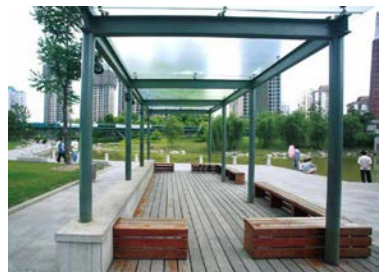
Simple structures that allow for hanging elements like sails and lights.
